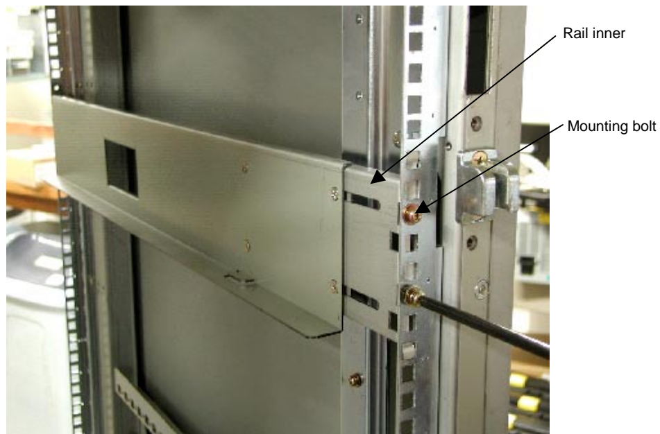
Figure 2-6. Securing the Inner Rail
